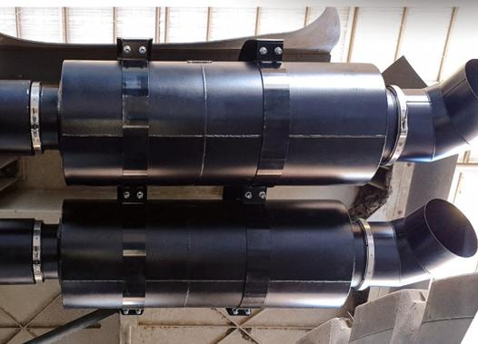
Dual-wall exhaust upgrades remove the need for thermal blankets on engine pipes
