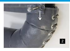
**OVERLAPPING SECTIONS** Blanket pieces should be fitted to overlap those in a position prone to gravity effects. This ensures liquids/fluid/debris runs off to remove seepage and potential ignition.
