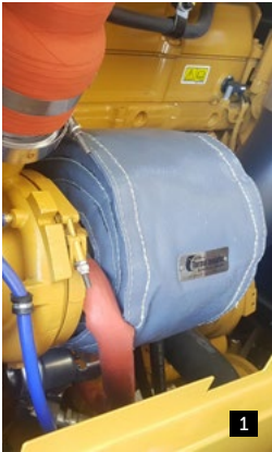
PHOTOS 1-7 Cat 24 manifold, turbo, e/pipe, muffer, t/pipe blankets
