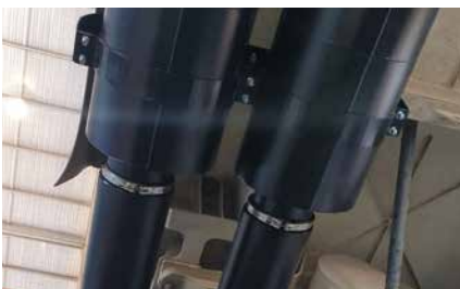
Dual-walled exhaust pipes remove the need for blankets and related maintenance
